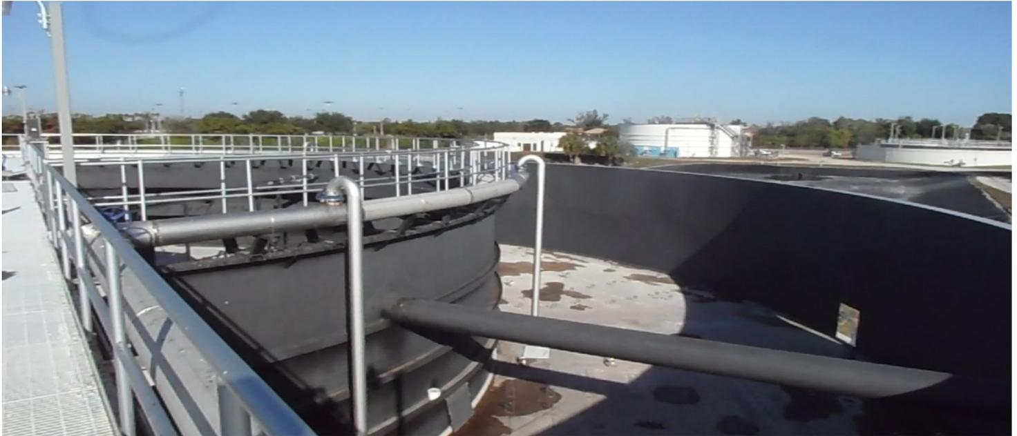
Above is the clarifier and digester section of a three-chambered 1.6 million gallon wastewater processing tank used for treating the inflow from the customers of the district. Once the process is complete the treated water will be injected 3,500 feet below ground as permitted for permanent disposal.
