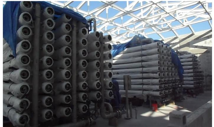
The construction progress photo above shows installation of three membrane "trains" and the high strength steel roof girders prior to the installation of the roof decking.
